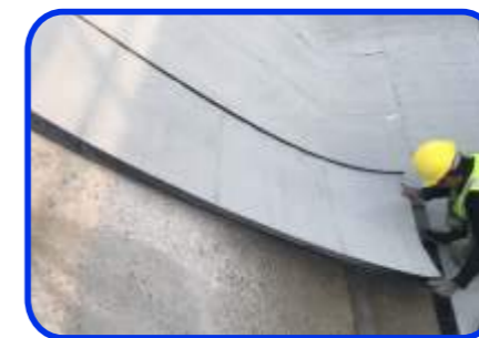
2. Membrane Installation
