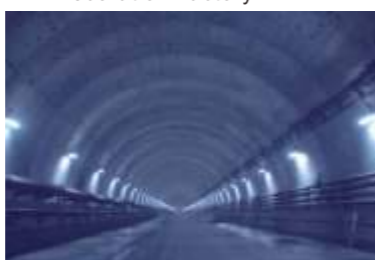
Nanjin Yangtze River Tunnel
