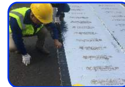
5. Trial Laying of Membranes & Marking
