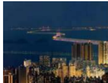
Hong Kong-Zhuhai-Macao Bridge
