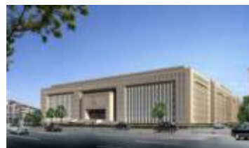
Office Building of China Ministry of Public Security
