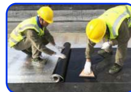
7. Paving the Membrane while Brushing the Rubber Bitumen Coating
