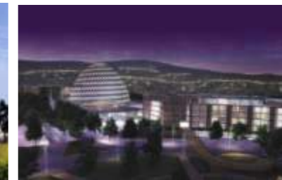
Kigali Convention Center -Rwanda, Africa
