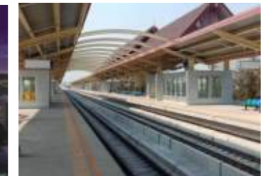
Double Track Railway Northeast Line -Thailand
