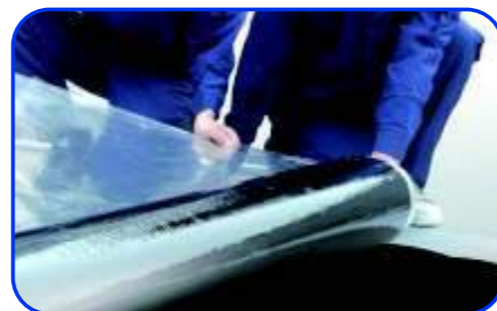
4. Paving of Waterproof Membrane
